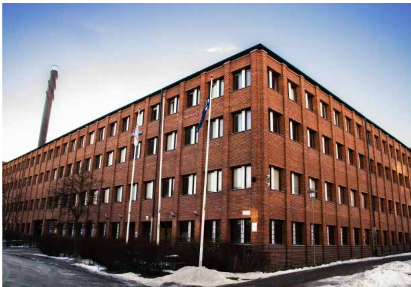
Vincero Fastigheter's property on Instrumentvägen 29-31 in Stockholm consists of offices and warehouses.
