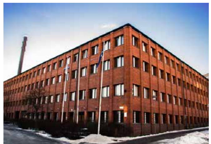
Vincero Fastigheter's property at Instrumentvägen 29-31 in Stockholm consists of offices and storage space.
